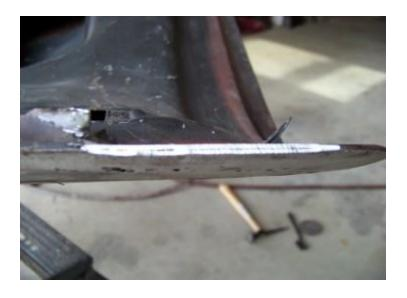
Take the grinder and grind the inside lip off the corners. Now using the pry bar and a hammer, tap the lip off the trunk lid. If you run into any resistance, stop and use the grinder to loosen any stuck areas.
